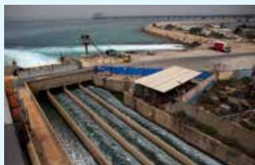
Brine water flows into the Mediterranean Sea after passing through a desalination plant. Photo by Nir Elias/Reuters
